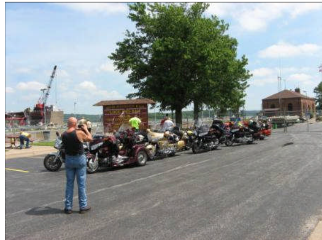
Lock and dam 16 in Illinois.
